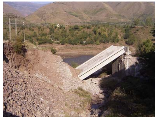
Fig. 23: Abutment failure of a bridge on Road No. 3, east of Muzaffarabad
