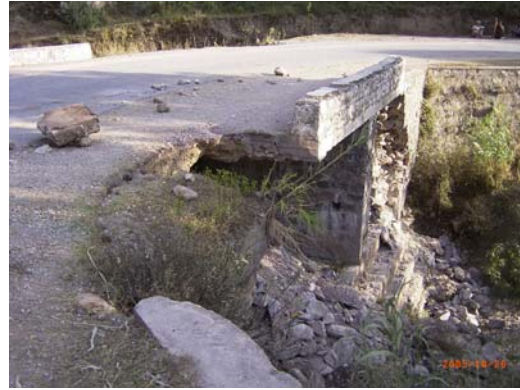
Fig. 21: Abutment failure of a bridge on a local road in south of Balakot
