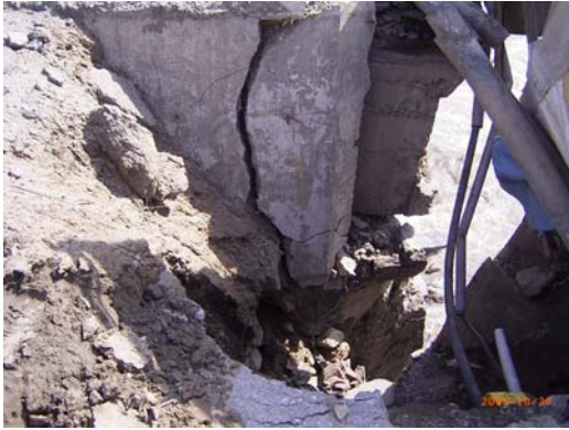
Fig. 20: Abutment failure of Balakot Bridge
