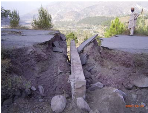
Fig. 22: Collapse of a culvert on a local road in south of Balakot
