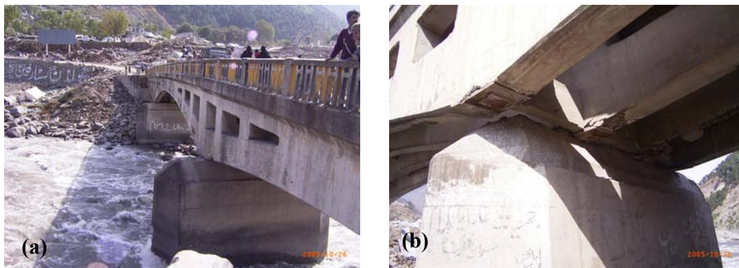
Fig. 19: Displacement of deck of Balakot Bridge towards south and east.
